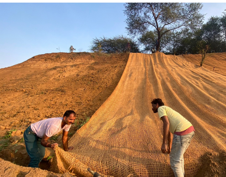
Installation of coir mat on contoured surface.
