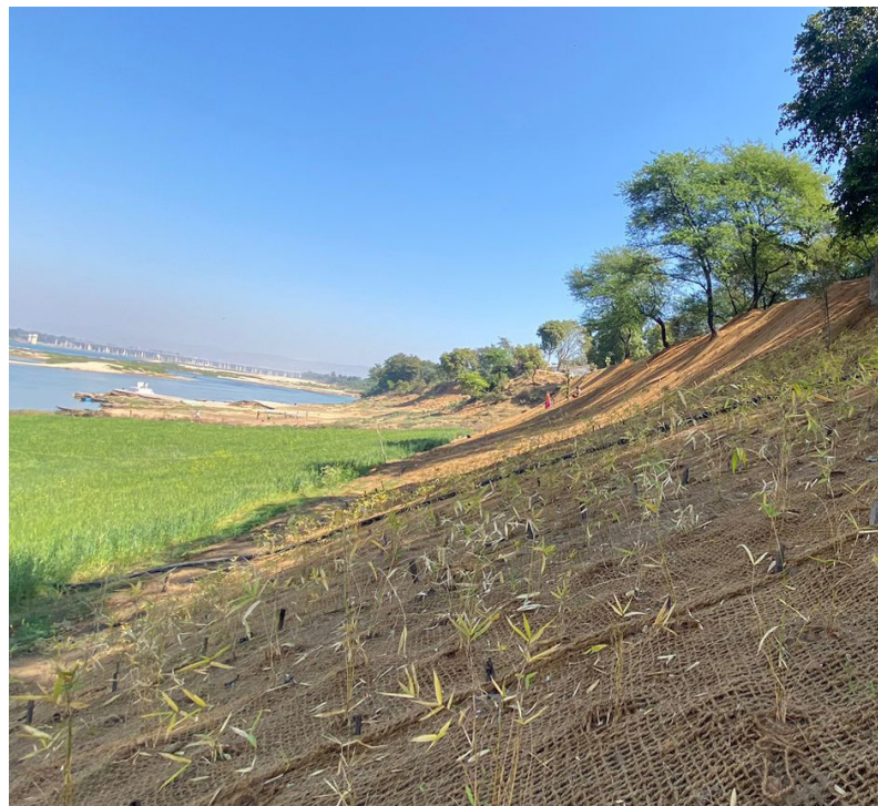
Slope stabilisation via bamboo combined with coir mat, with cultivation above and below.
